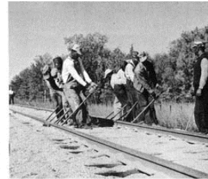
A track lining crew in Alabama, with the caller on the right and the white section boss in the distance
